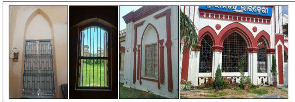
Figure 14:Various Types of Metal Grills used in the openings
