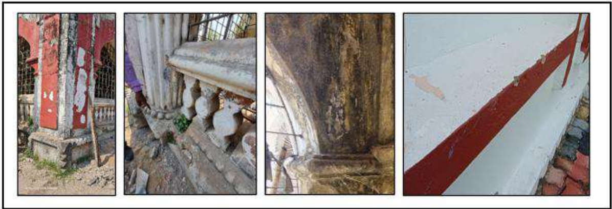
Figure 8: Plaster deterioration
