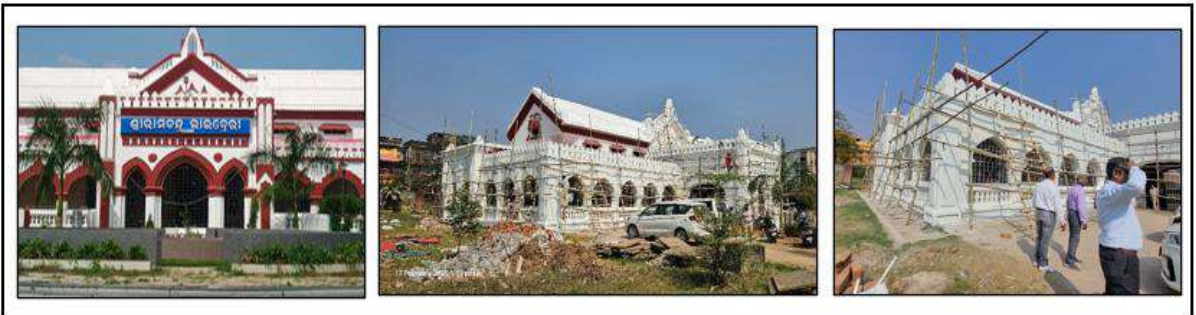
Figure 9: White putty treatment on the surface topped with plastic paint
