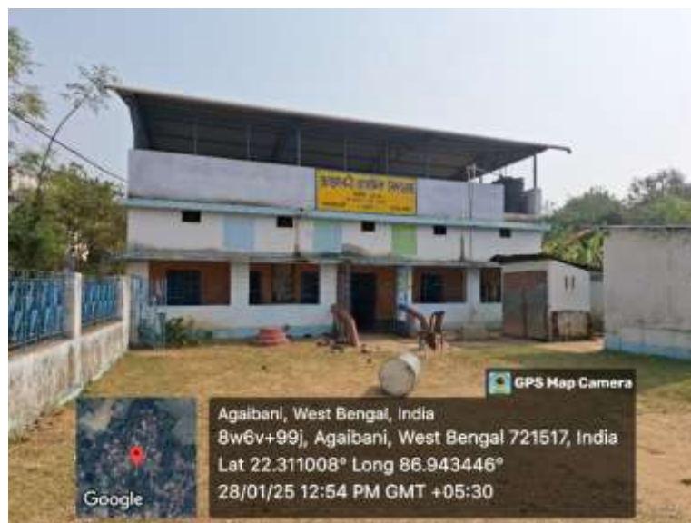
Figure 3.22 Aguibani Primary School
